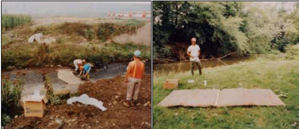
Plate 4-8 Typical Sedimat Details (Source: https://www.hy-tex.co.uk/ ).
