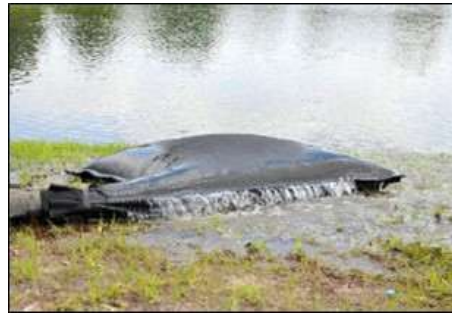
Plate 4-7 Silt bag under inspection
