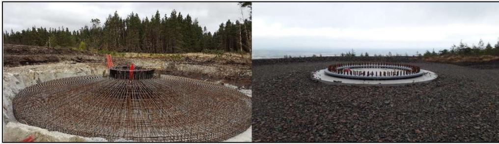
Plate 4-2 Turbine 'Anchor Cage' and finished turbine base
