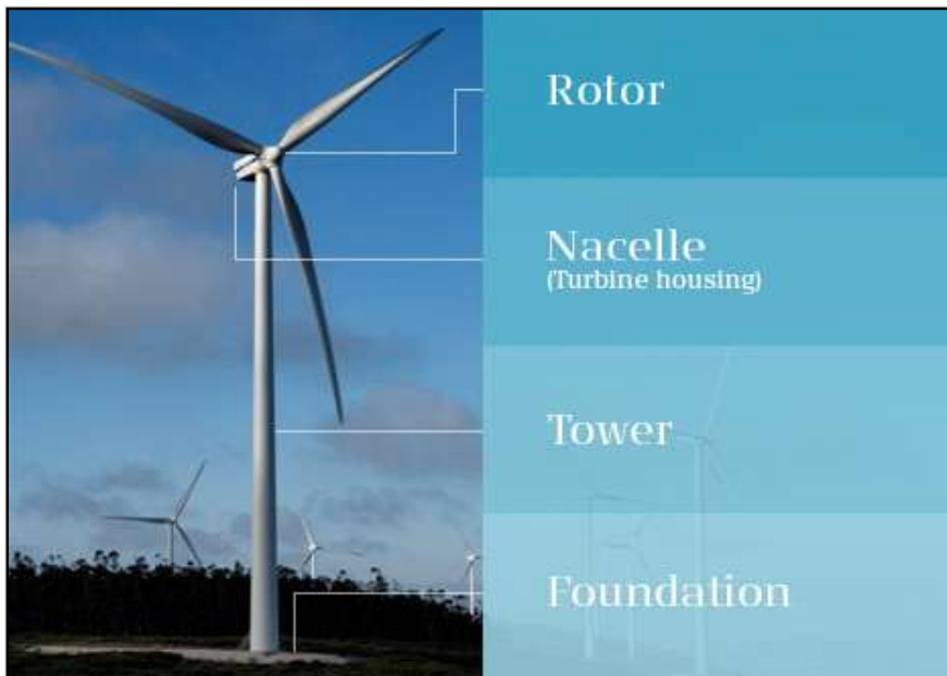
Plate 4-1 Wind turbine components
