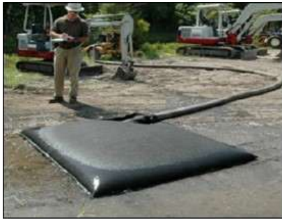
Plate 4-6 Silt bag with water being pumped through
