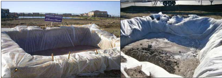
Plate 4-3 Concrete washout area
